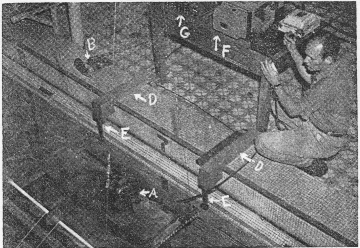
FIGURE I. Towing Apparatus, Measuring Device, and Pacing Device. Key: A. Motor; B. Placing device; C. Step pulley; D. Iron clamps; E. Steel beams; F. MRC Strain Gage Control Unit; and G. Hathaway S14-C Galvanometer.
